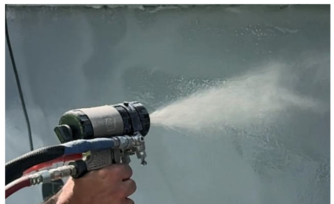
Wall application with two-component spray equipment
