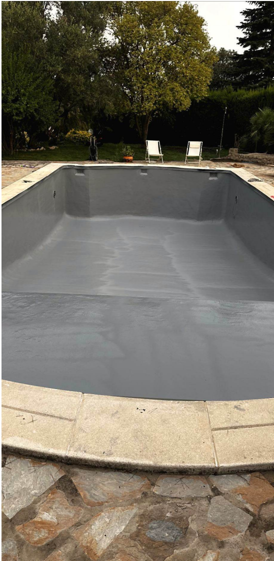
Seamlessly applied membrane, ready for the topcoat
