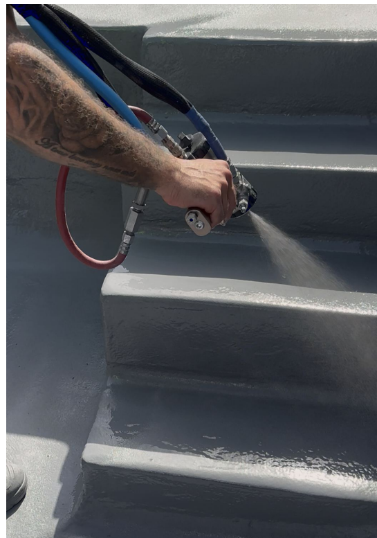
Application on the steps: layer by layer up to the required thickness
