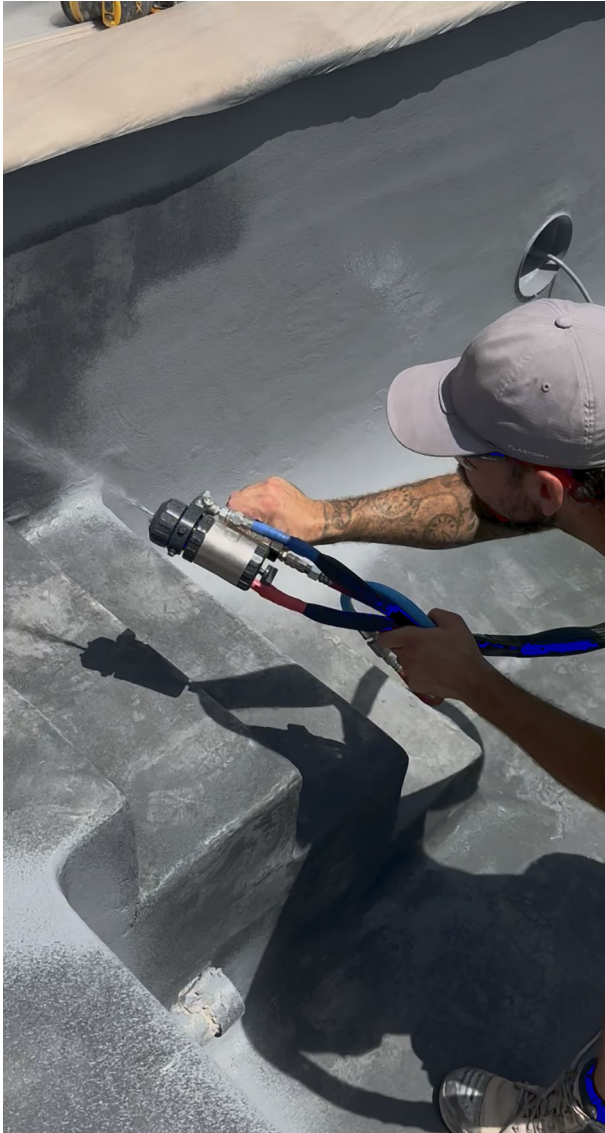
Application of the membrane in the corners and curves
