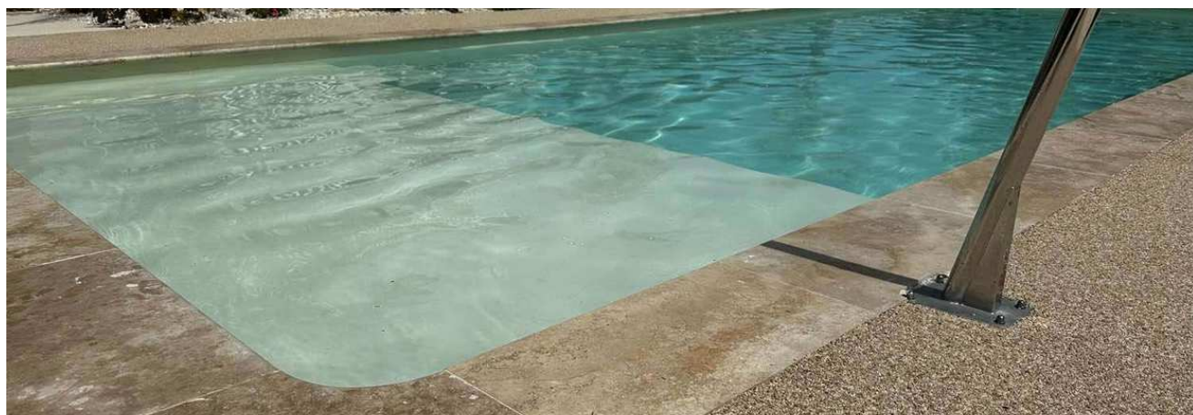
— The travertine edge and the chrome shower of the completed pool
